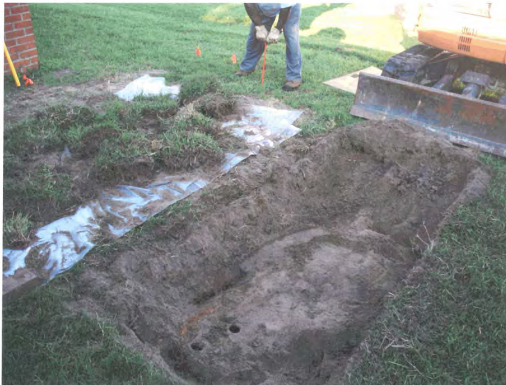
Picture 3: Excavation in progress on 745Bluebell-3.
