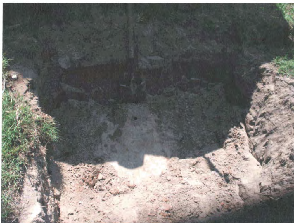
Picture 2: Excavation in progress.
